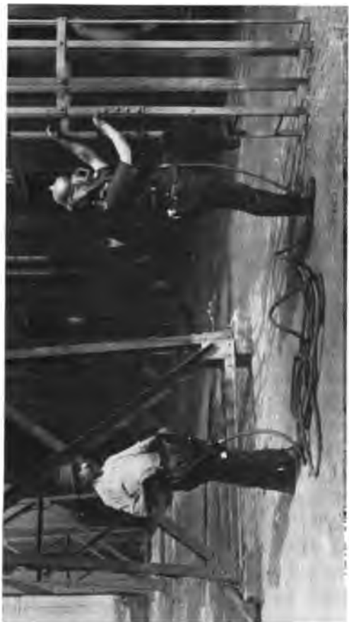
Fig. 2. Helmet, with Hose Connection and Bellows for supplying Fresh Air.†
